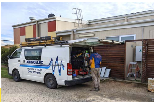
JohnoElec install the batteries
