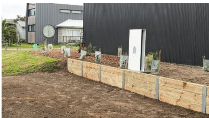
Site prepared for EV charger beside Men's Shed
